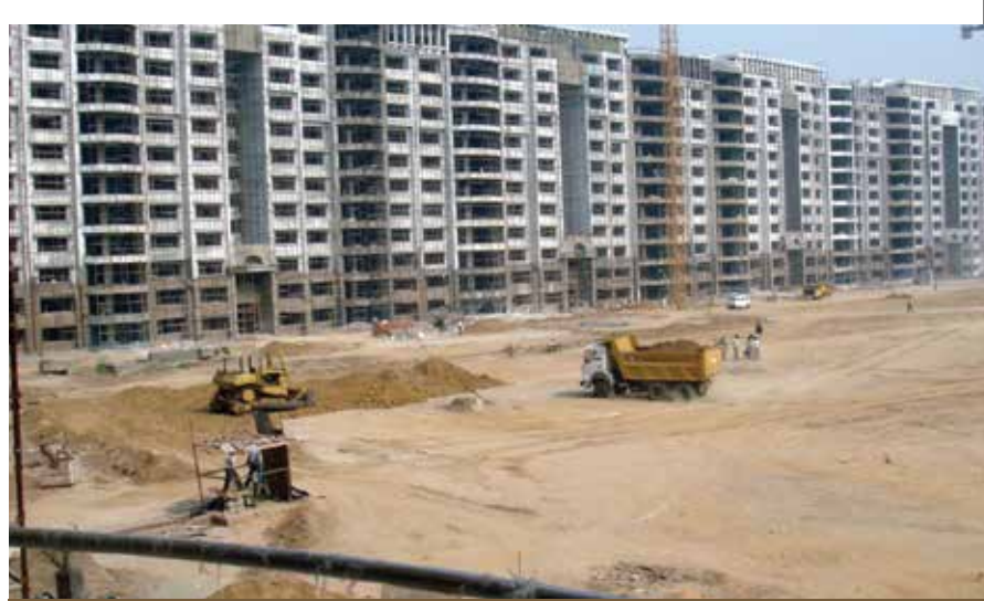
Site clearance and start up
