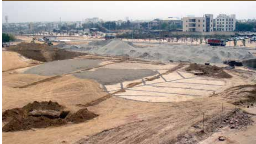
Drainage, sand capping and pump house excavation
